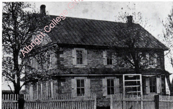
DREISBACH'S HOME NEAR LEWISBURG, PA.
