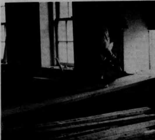
Construction worker planing 2 x 4's on the second floor of Teel Hall. Renovations are expected to be finished by September. photo by Neil Lesitsky
