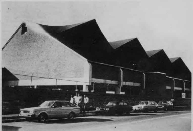
The unfinished Lifesports Center was dedicated last Saturday and remained open for the day's activities. The Center will now remain closed until work is completed.
