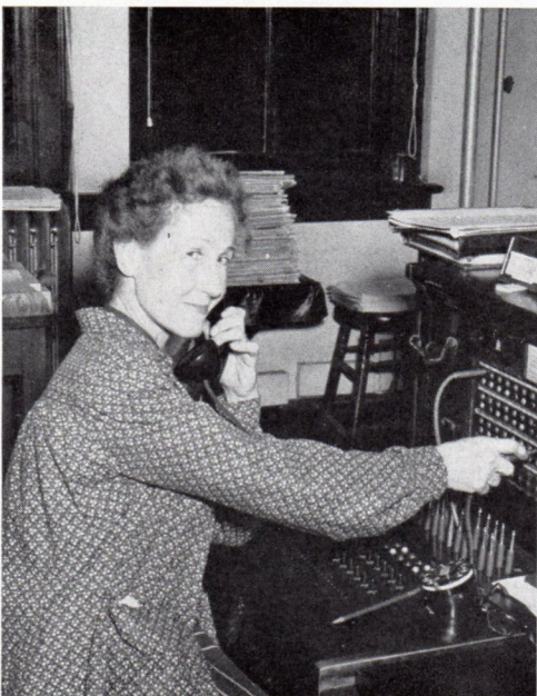
Switchboard MRS. ANNA S. ECK, Switchboard Operator
