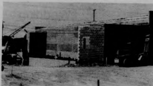
The new shopping center being constructed at the corner of 11th and Rockland Streets will contain a Giant supermarket and a Rite-Aid drugstore.
