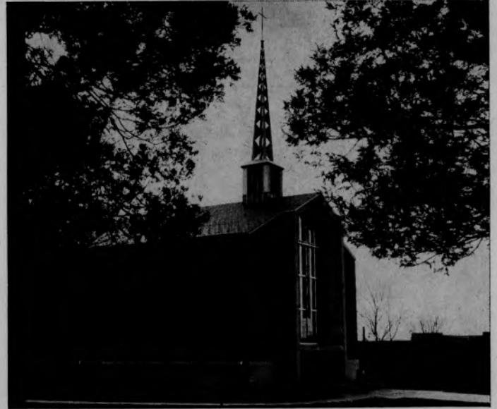
Dedicated in February, 1960, the Merner-Pfeiffer-Klein Memorial Chapel-Auditorium accommodates 925 for religious and cultural programs. Two faculty offices and four classrooms are on the ground floor.
